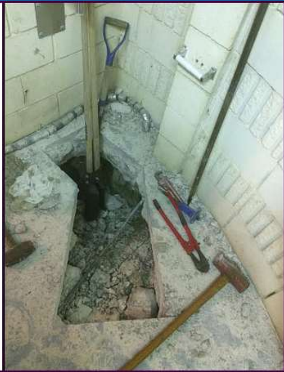
Removing Dirt and Rock
