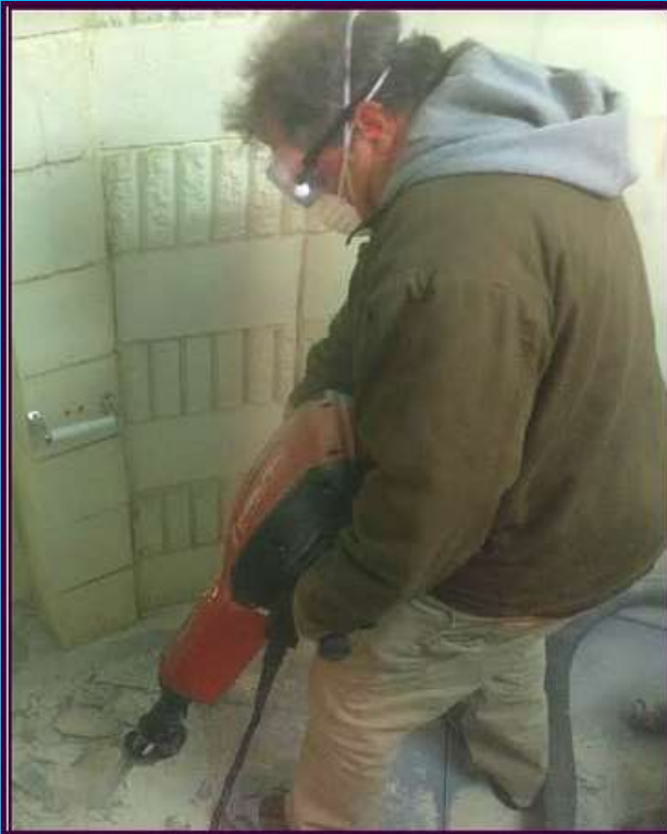
John Newton breaking up cement
