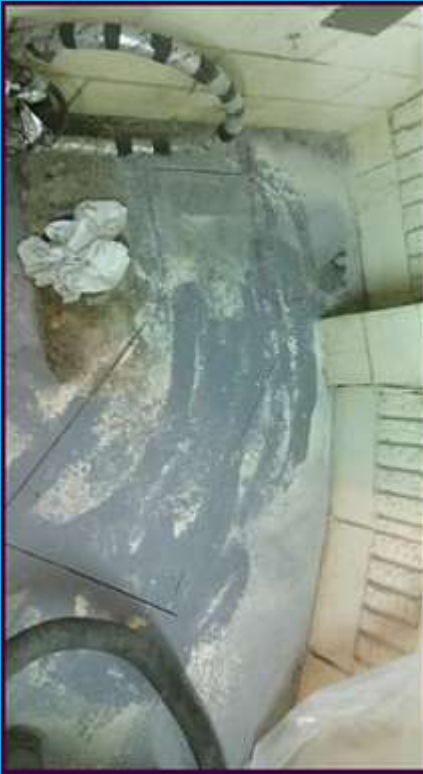
East Wall Before cut
